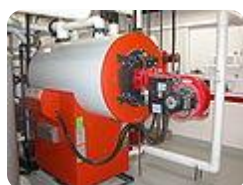
Condensing boiler
