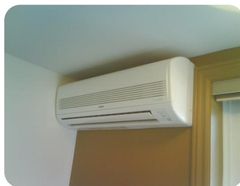
Indoor unit of a split air-conditioner
